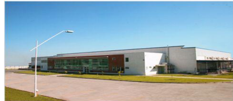
San Bernardo New IC Plant
